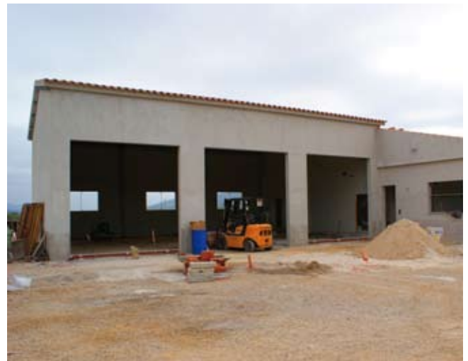
Construction work is ongoing for the Rural Emergency Brigade Base.
