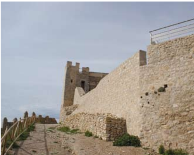
Restoration work continues at the Castillo de Xivert.
