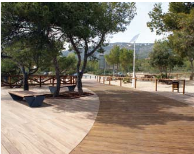
Final stretch of the Coastal Path finished.
